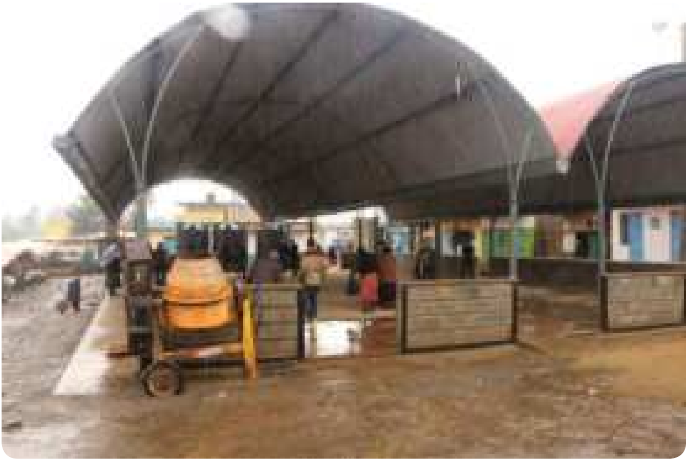
Construction of Njabini market
