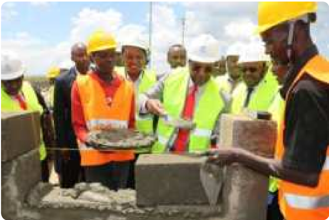
HE The Governor laying the foundation of the County Assembly administration block.
