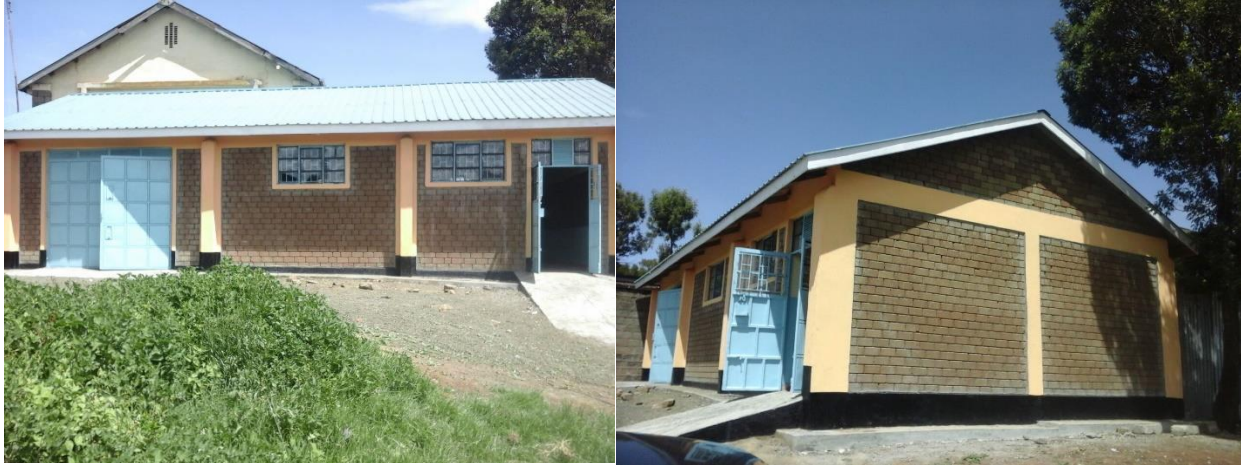
Plate 3.2: Appropriate Building Technology Centre in Molo
