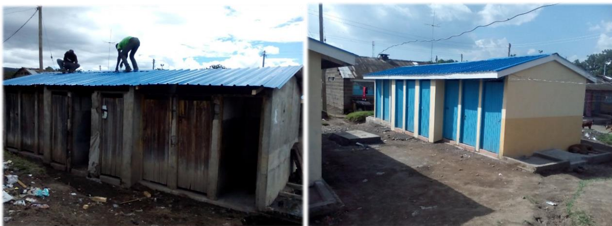
Plate 3.1: County Estates' face-lifting in Kimathi
