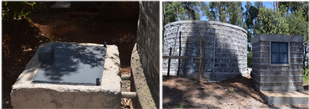
Plate 3.7: Water Project in Kuresoi North
