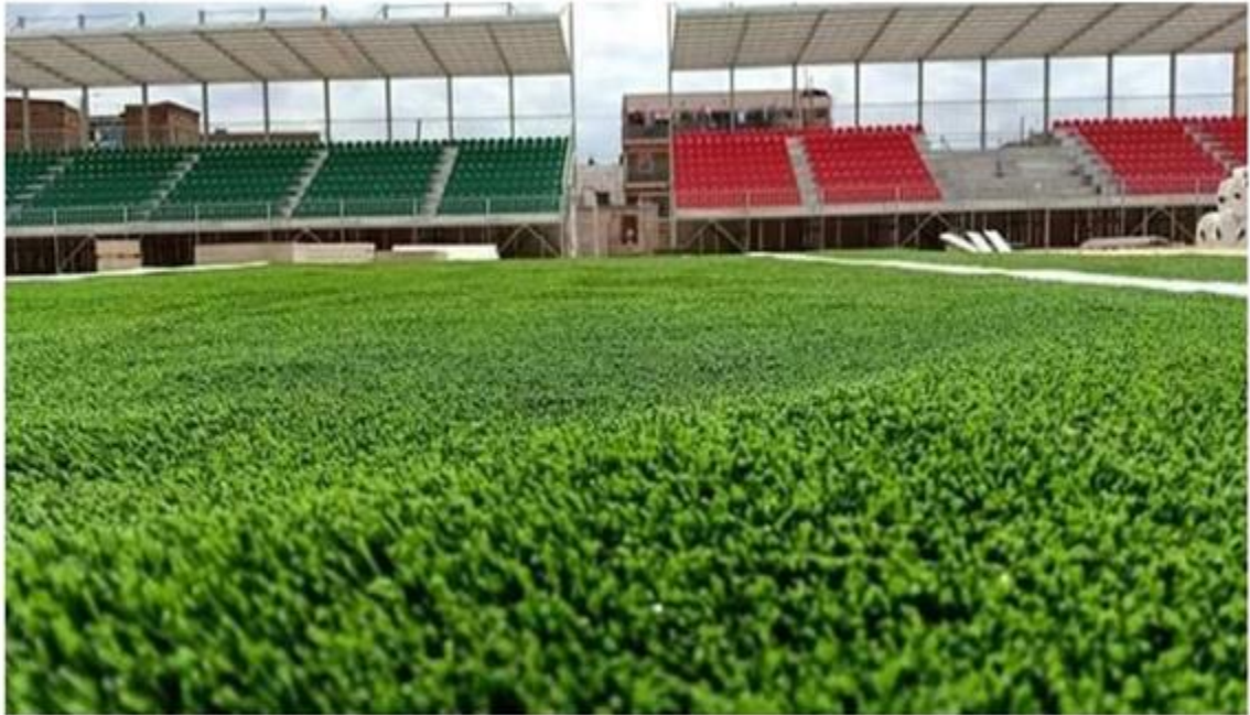
Ongoing Stadium at Dandora
